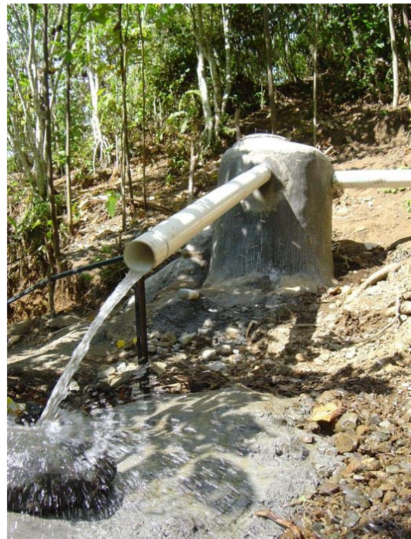
Sedimentation chamber with overflow back into the main creek
