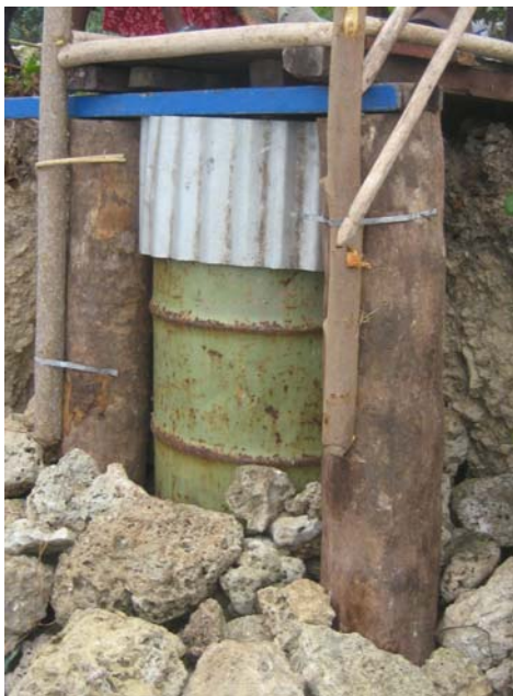
Figure 2. Collect information about current sanitation facilities and hygiene practices in target communities
